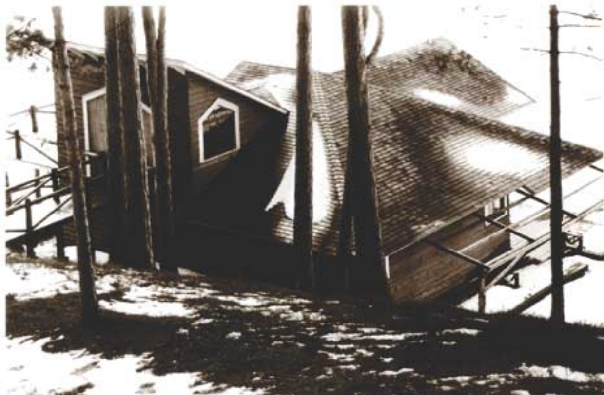
The roofline of the boat house from above.
