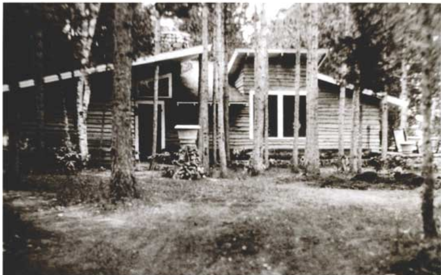
The main facade at White Pine was ahead of its time in terms of massing and use of angles. Its "brainstorm siding," milled weatherboarding with unsawn edges, was a rustic idiom credited to builder Ben Muncil, who pulled its name from the headlines of a scandal.
